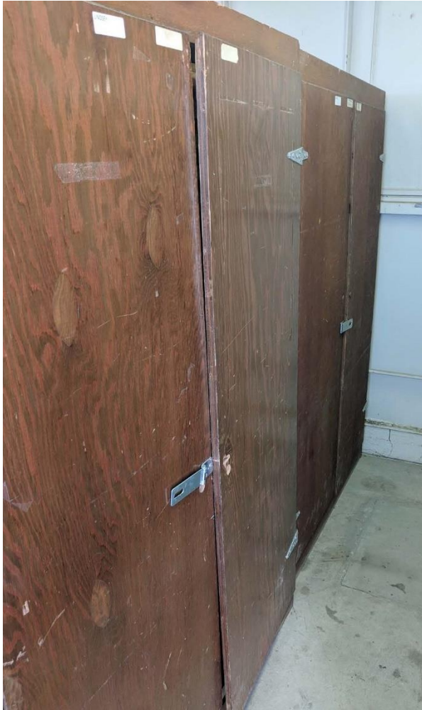
FIGURE 1. Old wooden cabinetry at the Desert Laboratory on Tumamoc Hill, out of alignment.
